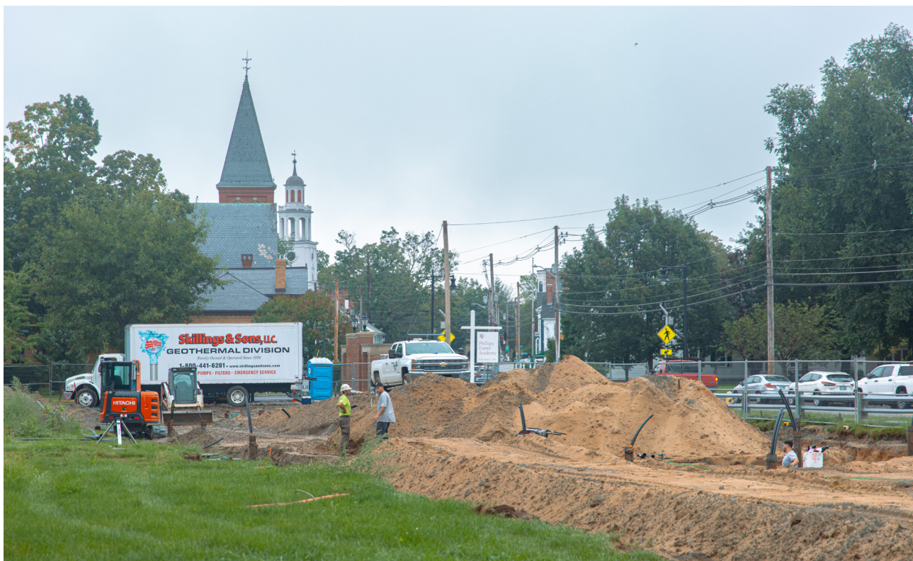
Geothermal wells are being installed on the Academy lawn.
